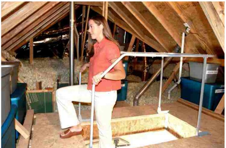
**Problem:** Entering or exiting the attic from a steep ladder is very dangerous without a hand-railing to hold onto and the unguarded ladder opening is a constant falling hazard while you are walking around and working in the attic!
